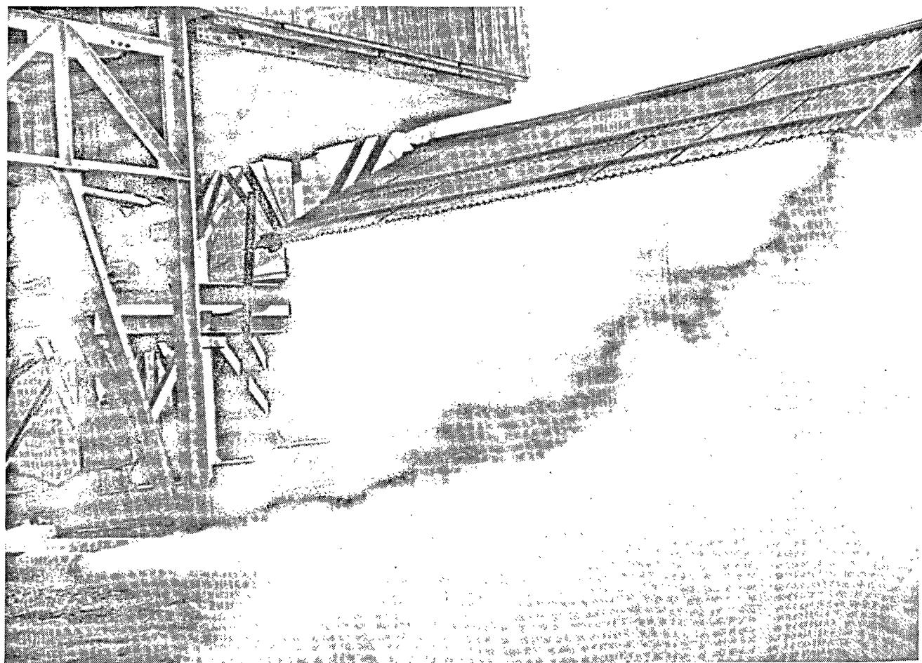
Figure 4. Air drilling (well discharge, as a dust cloud formed by air stream and powdered cuttings)
