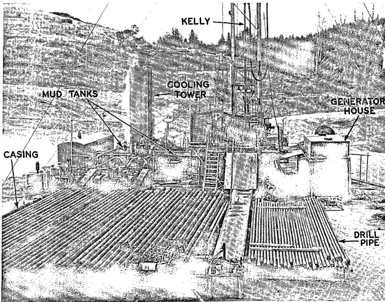
Figure 5. General layout at T 12 rig
