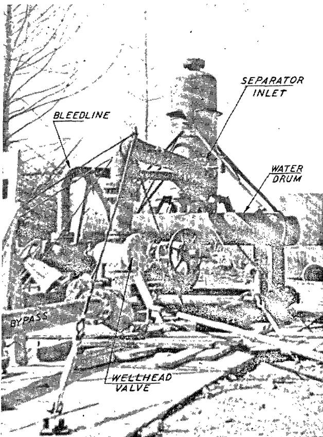
Figure 4. Test equipment
