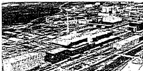
The Thermal Oxide Reprocessing Plant (THORP) in UK. This commercial process recycles spent fuel from UK and overseas reactors, separating the long-lived waste from uranium and plutonium. The smaller black building on the right is the ventilation plant for the waste.
