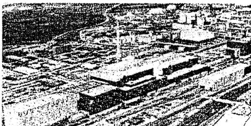
The Thermal Oxide Reprocessing Plant (THORP) in UK. This commercial facility treats spent fuel from UK and overseas reactors, separating the high-level waste from uranium & plutonium. The smaller black building on the right is the ventilation plant for the waste.
