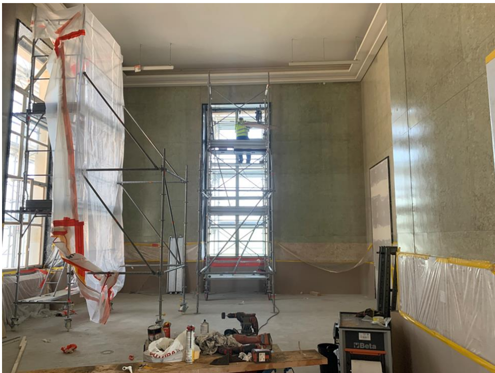
Figure IV Interior progress photograph showing renovation of windows in building AC, June 2021
